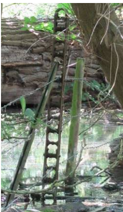
Late C19/early C20 iron stock fencing adjacent to White Brook south of gravel extraction bridge: post for strained wire (left); park rail style (centre); another style of post for straining wire, on boundary with willow plantation (right). These probably date from the Astor ownership.
